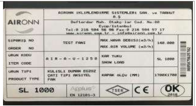
Description: Identification Plate of Actuated Cabinet Roof Type Axial Smoke Exhaust Fan
