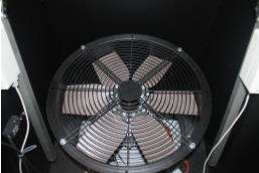
Description: General view of Actuated Cabinet Roof Type Axial Smoke Exhaust Fan
